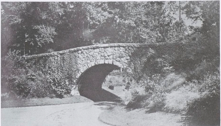
BRIDGE ON NORTH DRIVE MACKAY ESTATE
