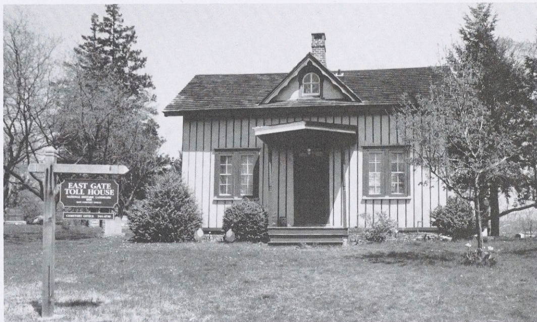
East Gate Toll House located in Roslyn Cemetery. Restored in 1976, it is the last remaining Toll House on Long Island. Photo copyright 1990 by Myrna Sloam; from the Bryant Library Local History Collection.
