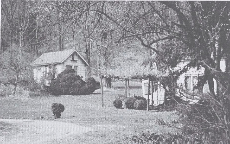
FORMER PRIVATE SCHOOL NOW BEHIND TARRANT HOUSE ON MAIN STREET
