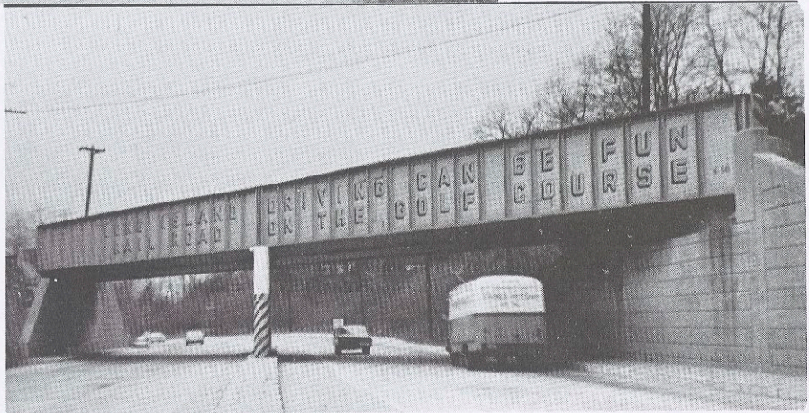
L.I. RAILROAD AT NORTHERN BLVD. 1962
