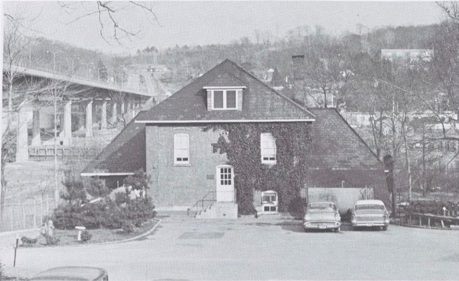
PUMPING STATION, ROSLYN WATER DISTRICT
